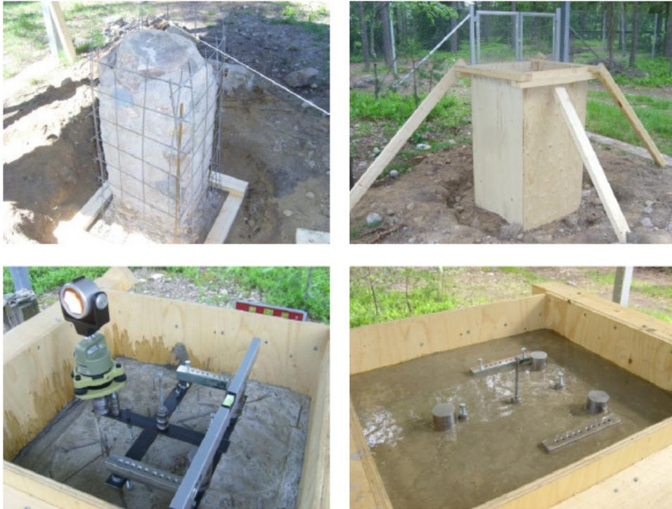
*Fig. 5. Reconditioning of the observation pillar at 24 m in June 2007. To maintain facilities for interference measurements, the new pillar-top structures had to be measured and installed exactly in their original places.*
