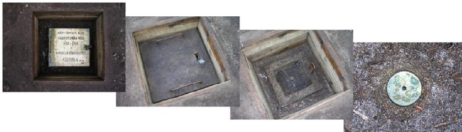
**Fig. 34.** The baseline lengths in the final results are the distances between the centres of the holes in the benchmark bolts of the underground markers, reduced to a reference height level.
