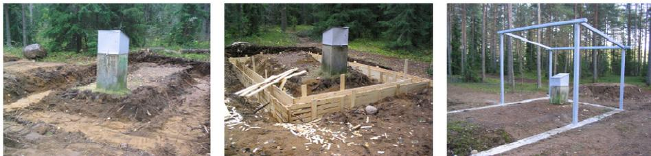
*Fig. 2. Protecting the underground markers and observation pillars in autumn 2004.*
