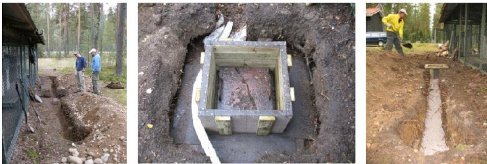
*Fig. 6. Installing a drainage system for the underground marker 0 in September 2007.*
